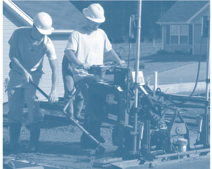
The Somero® Mini Screed™ is ideal for screeding residential and small commercial slabs on grade.
